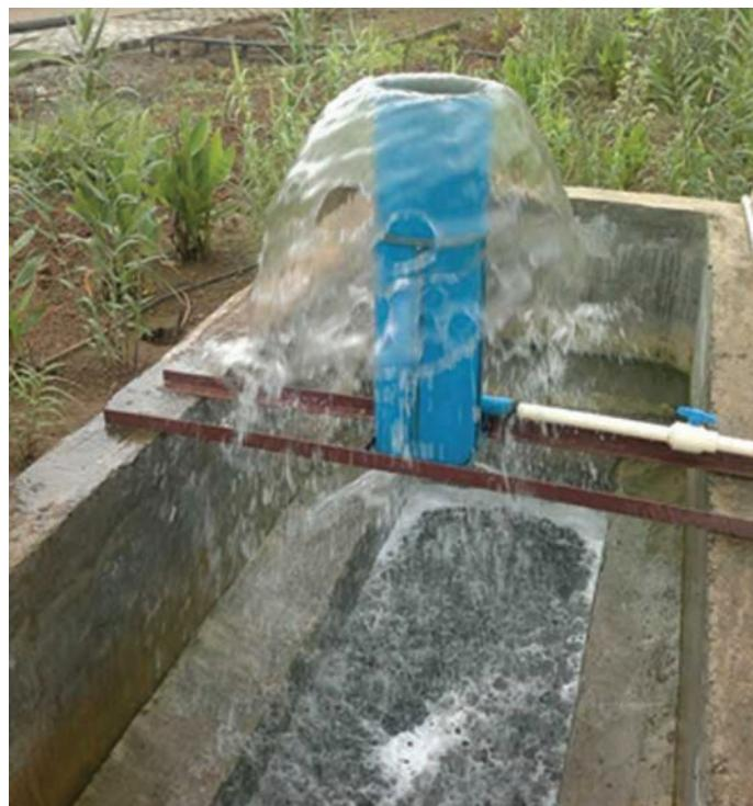
**Figure 4: Vortex Placed on the Polishing Pond Improved the Efficiency**
