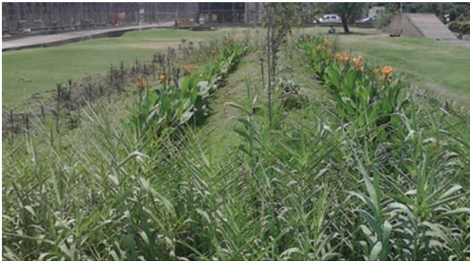
**Figure 3: Reed Bed System That Got Overloaded**
